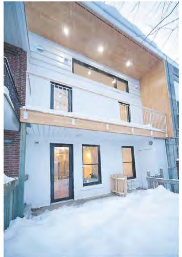
At the back, the cantilevered roof was renovated and the balcony on the third floor is sleeker and lets more light in.
